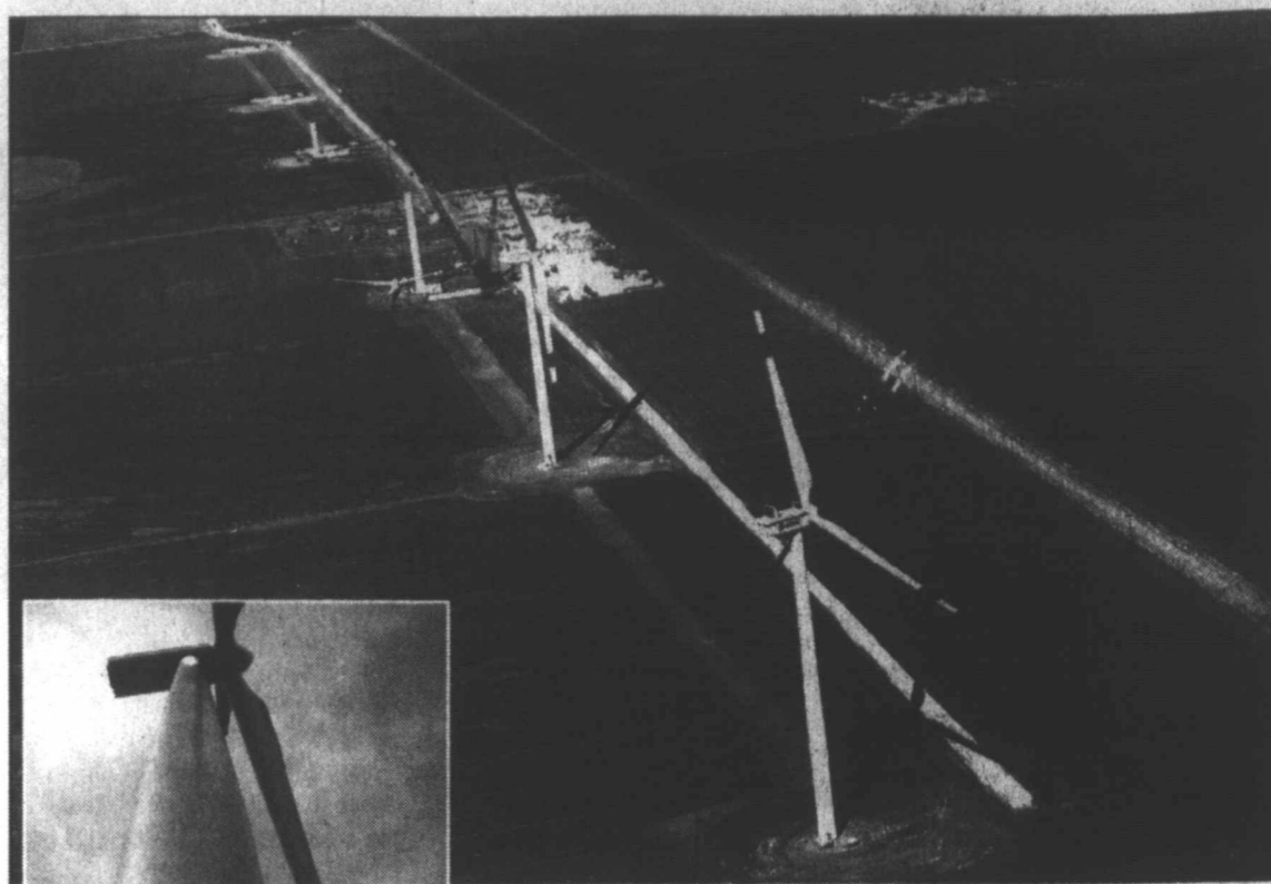
The view from above (and below) ... The photo above shows an aerial view of the Cirrus 1 wind energy project in southern Lynn County that was taken a week ago, showing the line of turbines running east and west, adjacent to County Road 32. Two of the 17 turbines were erected, and two more had lower tower sections in place. The other photo shows the view from underneath one of the completed turbines.
