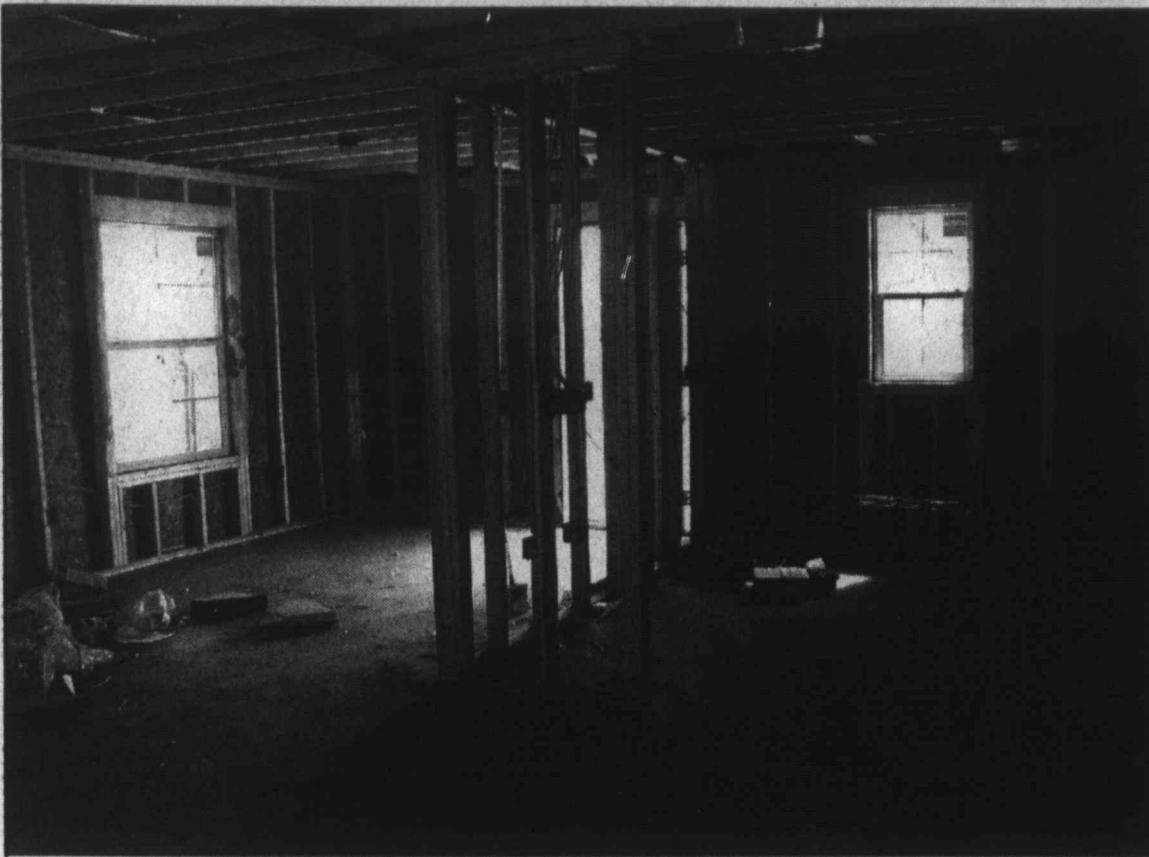
Coming together ... Two new houses under construction in Tahoka are coming along, featuring the exact same floor plans, part of a Texas Dept. of Housing and Community Affairs grant program that provides free homes to qualified applicants.
