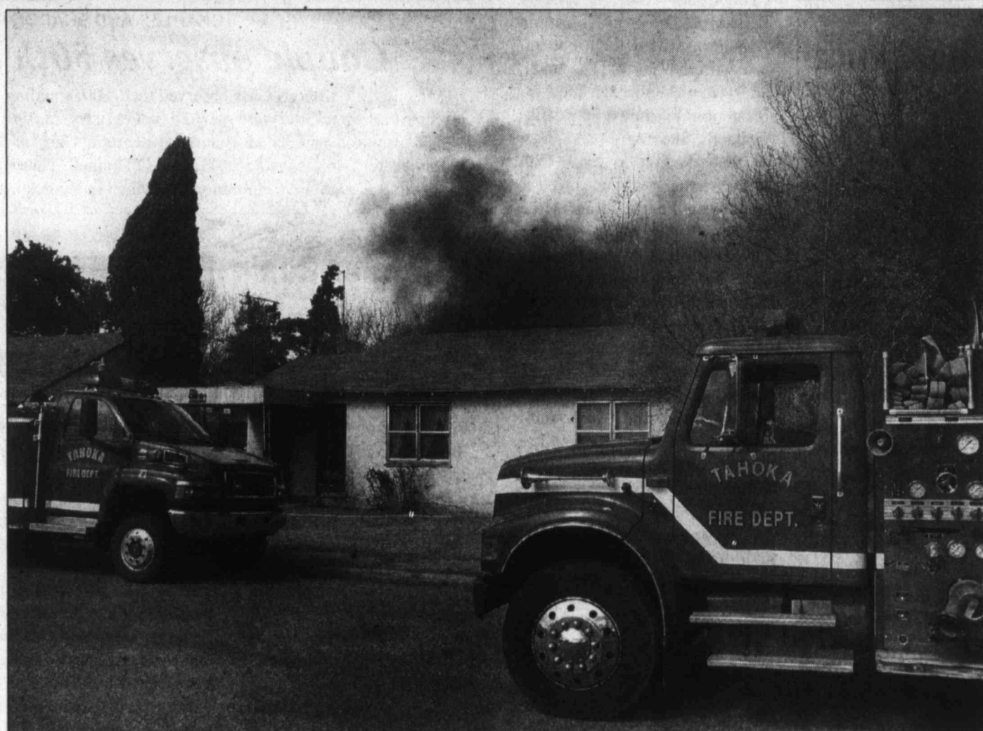
Fire does damage ... Tahoka Volunteer Fire Department responded to a fire alarm last Thursday at 2 p.m., arriving at the Hope Toscano home at 1708 N. 1st Street to see smoke billowing from a shed on fire in the back yard of the home. The fire damaged a bedroom on the back side of the house, and damaged two sheds in this yard and two sheds in the adjacent yard, at 1716 N. 1st, home of Mr. and Mrs. Todd Henry. The fence between the properties also was burned, and electrical lines were burned. Red Cross was contacted for the Toscano family, who reportedly had no insurance. Cause of the fire was undetermined, according to the City Fire Marshal.
