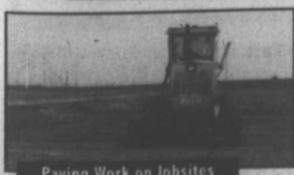
Paving Work on Jobsites
