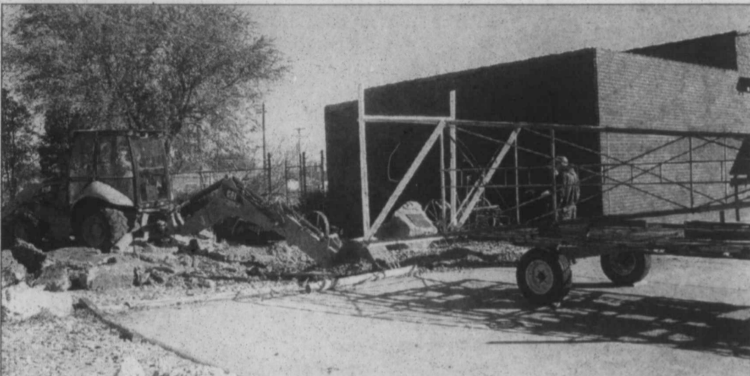
A New Old Windmill... It's an old windmill, but it's a new attraction at the Tahoka Pioneer Museum. Workers are digging holes for the legs of the metal tower which is being donated by Joe Don Nevill as a replacement for the old wooden windmill which formerly was placed just west of the museum on Lockwood. The older wooden structure had to be taken down because it was deteriorating and posed the threat of falling. Nevill said the metal windmill, still typical of many early-day windmills in the area, will be safer and easier to maintain. (LCN PHOTO by Pam Elrod)
