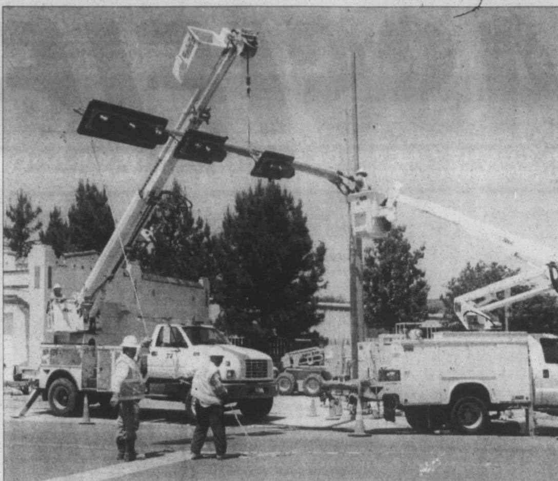
New traffic lights... New traffic lights were installed in Tahoka recently at the intersection of Lockwood (U.S. Hwy. 380) and Main. City officials and local TxDOT representatives could not offer any information on the lights, except to say that the state had contracted to replace the lights. The new lights are erected on poles over the street, replacing the lights that hung from lines crossing over the intersection (although the old lights are still working until the new ones are operational). (LCN PHOTO)
