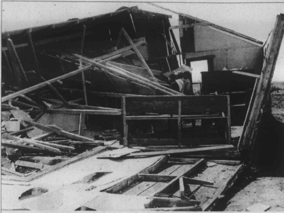
1957 Tornado Damage ... The tornado that hit on graduation day, May 24, 1957, completely destroyed the Antioch Baptist Church in Tahoka, leaving only the upright piano standing. That week's issue of The Lynn County News reported that two boys were seen playing the piano shortly after the storm passed.
