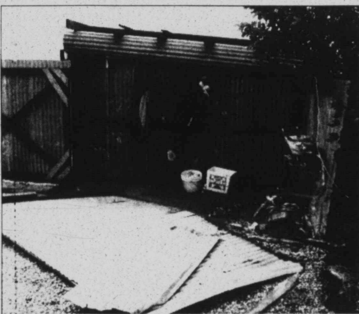
High winds rip walls from cart house ... Several golf cart houses were damaged by storm winds at T-Bar Golf Course Saturday, when an afternoon thunderstorm struck the area. This cart house still has a couple of walls standing, but five other houses were completely destroyed, and several other cart houses were damaged. (LCN PHOTO by Gary Jones)
