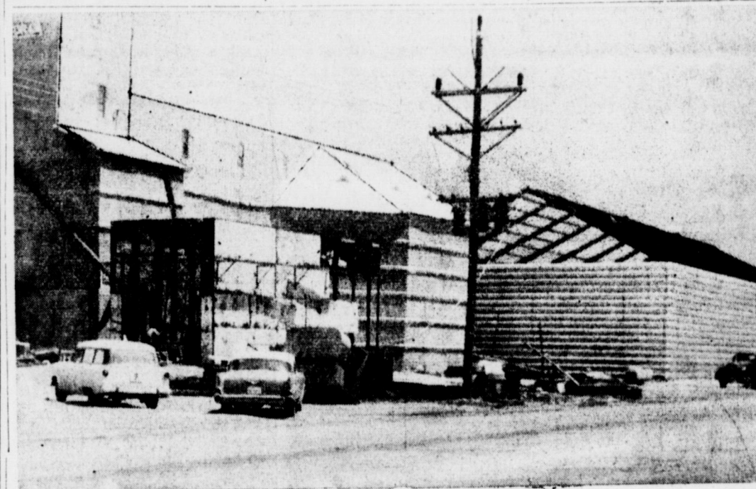
MORE MULESHOE BUILDING . . . The storage space that will bring the total Muleshoe Elevator Cooperative is completing an addition to their already large
