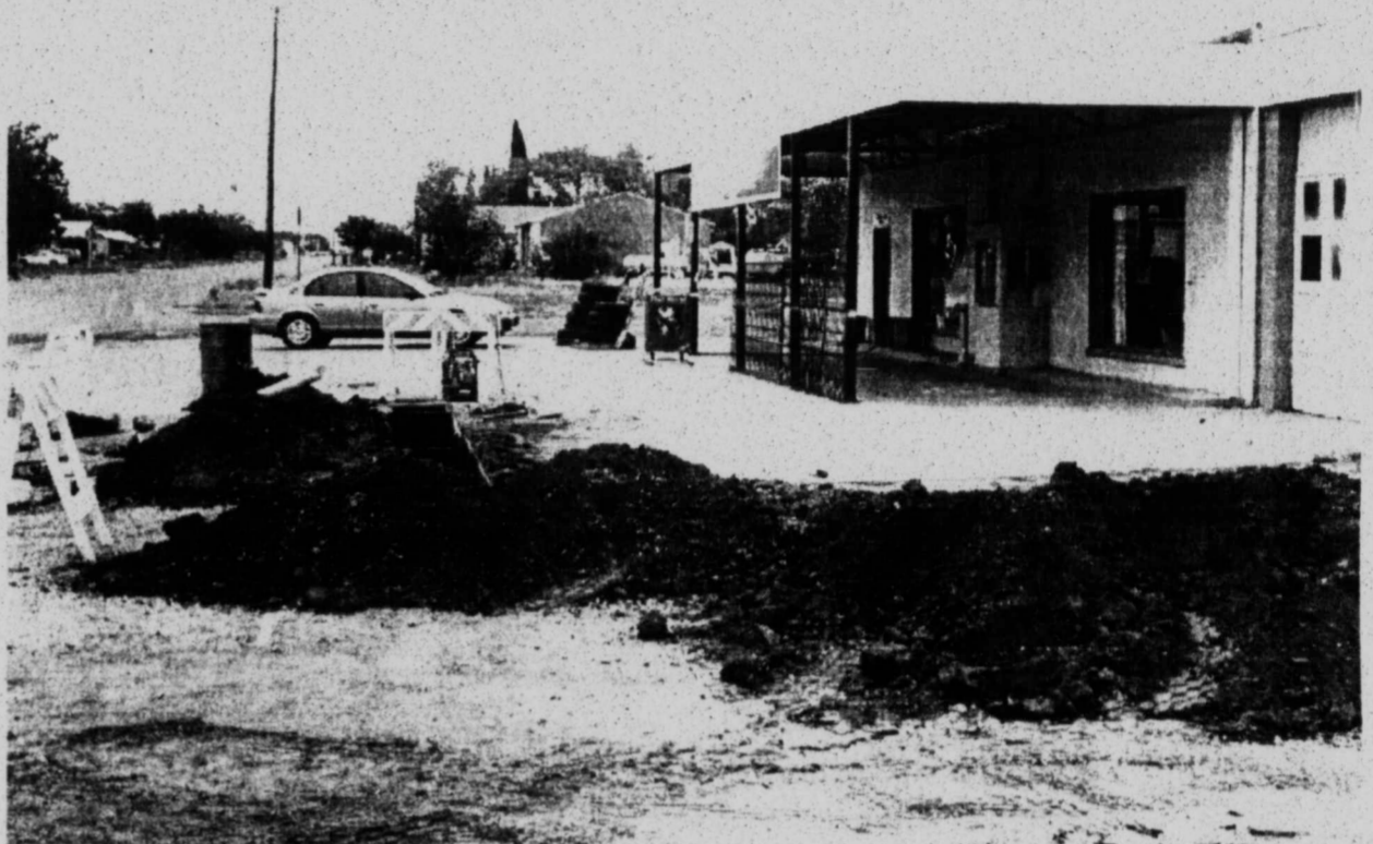
BIG GOPHERS? - Mounds of dirt surround Fuzzy's Station in Tahoka as the Texas Environmental Quality Commission digs to check wells. (LCN PHOTO)
