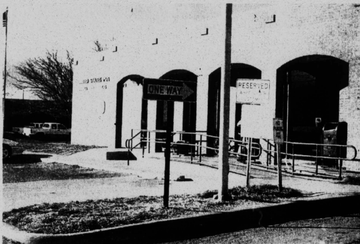
NEW ONE WAY DRIVE-THRU - The paved area between the U.S. Post Office and First National Bank in Tahoka has new one-way signs in place, and motorists are encouraged to observe the new one-way drive-thru. After the first of the year, according to Postmaster Kent Bartlett, the outside mail box will be moved to curbside to allow motorists to place outgoing mail in the receptacle from their cars. Parking will no longer be allowed in this area, Bartlett says, to accommodate the drive-thru mail box. (LCN PHOTO)
