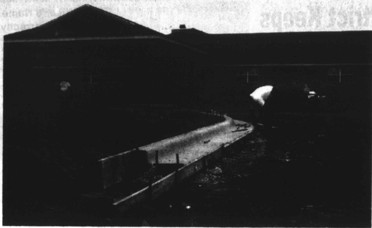
LYNNWOOD DRIVE —Workers last week poured curbs preparatory to putting in a driveway for the new Lynnwood Assisted Living Center next to Lynn County Hospital. The 20-unit facility is expected to be finished late this month. (LCN PHOTO)
