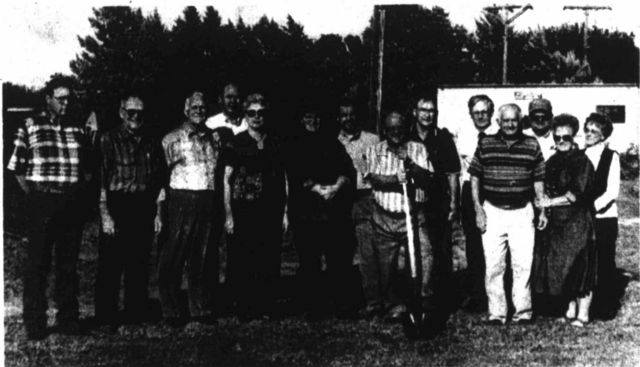
GROUND BREAKING CEREMONIES - Lynn County Hospital District had groundbreaking ceremonies last Wednesday afternoon for their new Assisted Living Center, to be built just north of the hospital. Construction of the new center, called Lynnwood, is expected to be completed in June 2001. Present for the groundbreaking were hospital board members, administrator, and doctors, as well as all four city mayors in the county. Shown from left are James Williams, mayor of O'Donnell, Jerry Ford, Administrator Dan Powers, Jackie Bishop, mayor of Wilson, Virginia Griffing, Peggy Morton, Dr. Griffith Thomas, Dalton Wood, Billy Tomlinson, Dr. Bruce Fried, Don Sharp, mayor of New Home, Mike Mensch, mayor of Tahoka, Lavonne Sharp, and Joy Brookshire. (LCN PHOTO)
