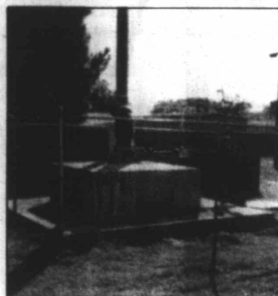
Water well improvements - City of Tahoka
