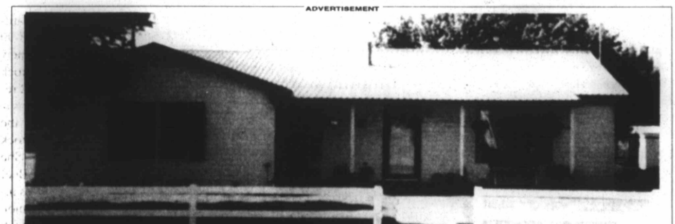
NEW STYLE —If your roof has been damaged or needs replacing after suffering hail damage, consider a permanent steel roof installed by Cover-All Home Pros. Recently installed steel roof and siding at the home of Wayne & Vickie Parker, 1201 S. 2nd in Tahoka, resisted baseball-size hail.
