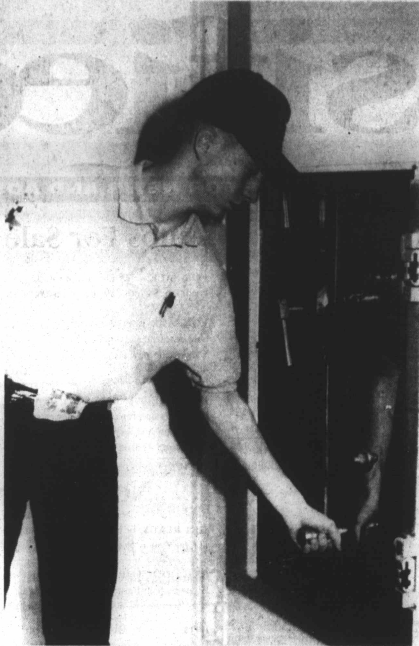
CLOSING MAXIMUM SECURITY DOORS - Lynn County jailer Mark Royce operates the mechanism for opening and closing the doors in the maximum security wing of Lynn County Jail. The small one-man cells can be opened and closed without any physical contact with the maximum security prisoners, and meals are passed through a small opening in each door. (LCN PHOTO)
