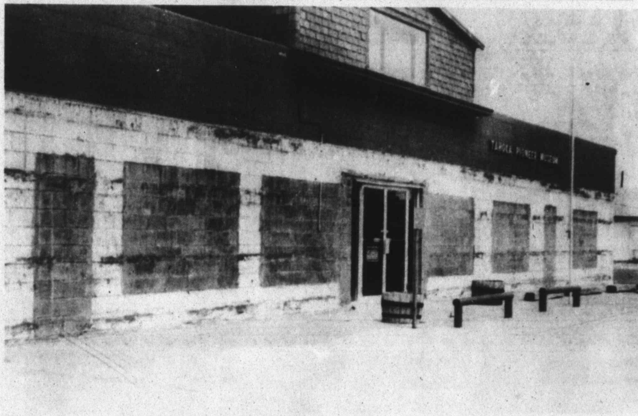
MUSEUM FACELIFT -- The Tahoka Pioneer Museum is in the process of being bricked. The old siding was rotting and instead of trying to replace it the Board of Directors decided to have the exterior bricked. (LCN PHOTO)
