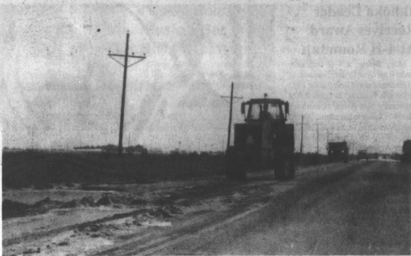
MOVING THE MUD - A highway department loader moves mud off FM 400 between Tahoka and Wilson one afternoon after the rains floated the topsoil onto the road. Several area roads were under water (and mud) for several days following the onslaught of rain during the past weeks. (LYNN COUNTY NEWS PHOTO)
