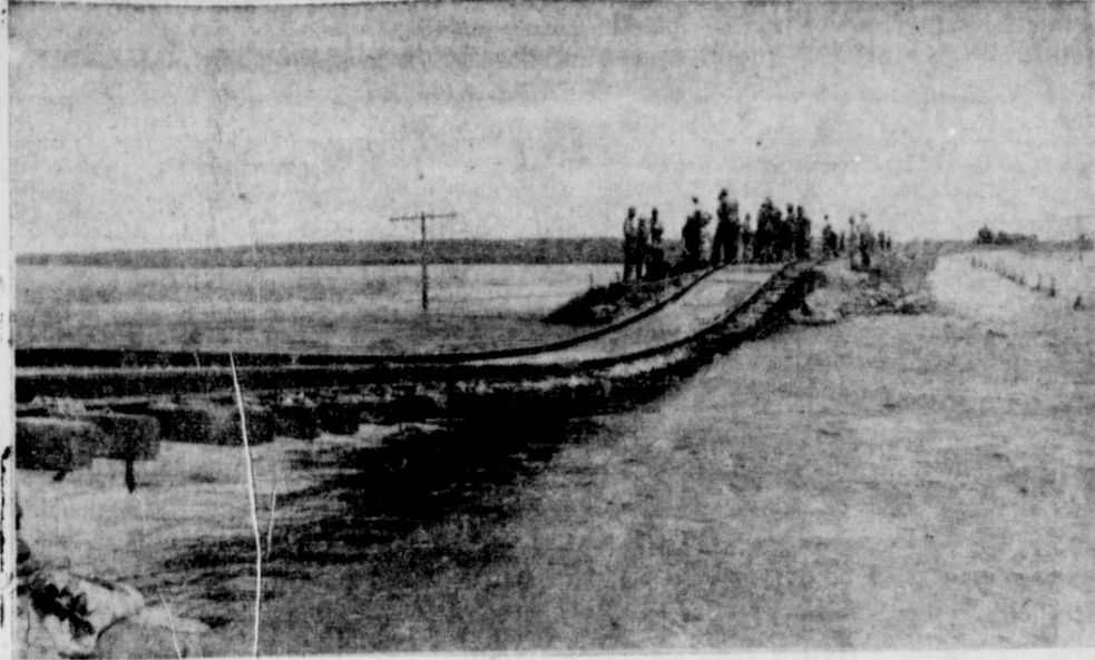
ACK IN '41 — folks used to have to walk across this railroad tie-bridge to reach the town on the other side. The inconvenience was caused by the great rains of 1941. Muleshoe measured 43.52 inches of moisture then and considerable flooding occurred, including this Santa Fe washout which prevented the "Chief" from reaching town. Photo by Muleshoe's past.
