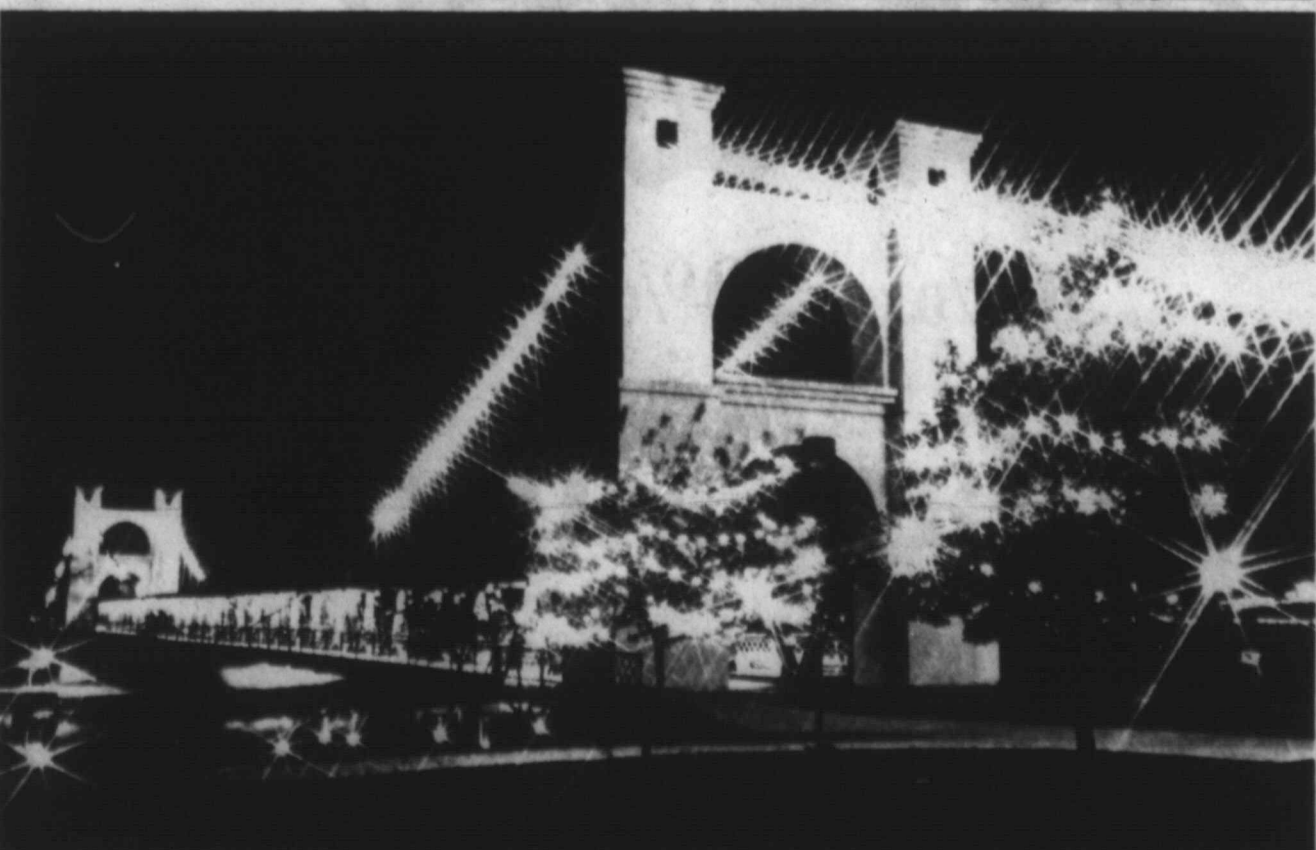
The Waco Suspension Bridge was the longest of its kind in the nation when it was built back in 1870. Thousands of cattle and numerous wagon trains passed over the structure in its heyday, and the famous Brooklyn Bridge in New York was patterned after it. The 475 ft. bridge is still used today, but only as a pedestrian crossing. Tourism Division, Texas Dept of Commerce photo.
