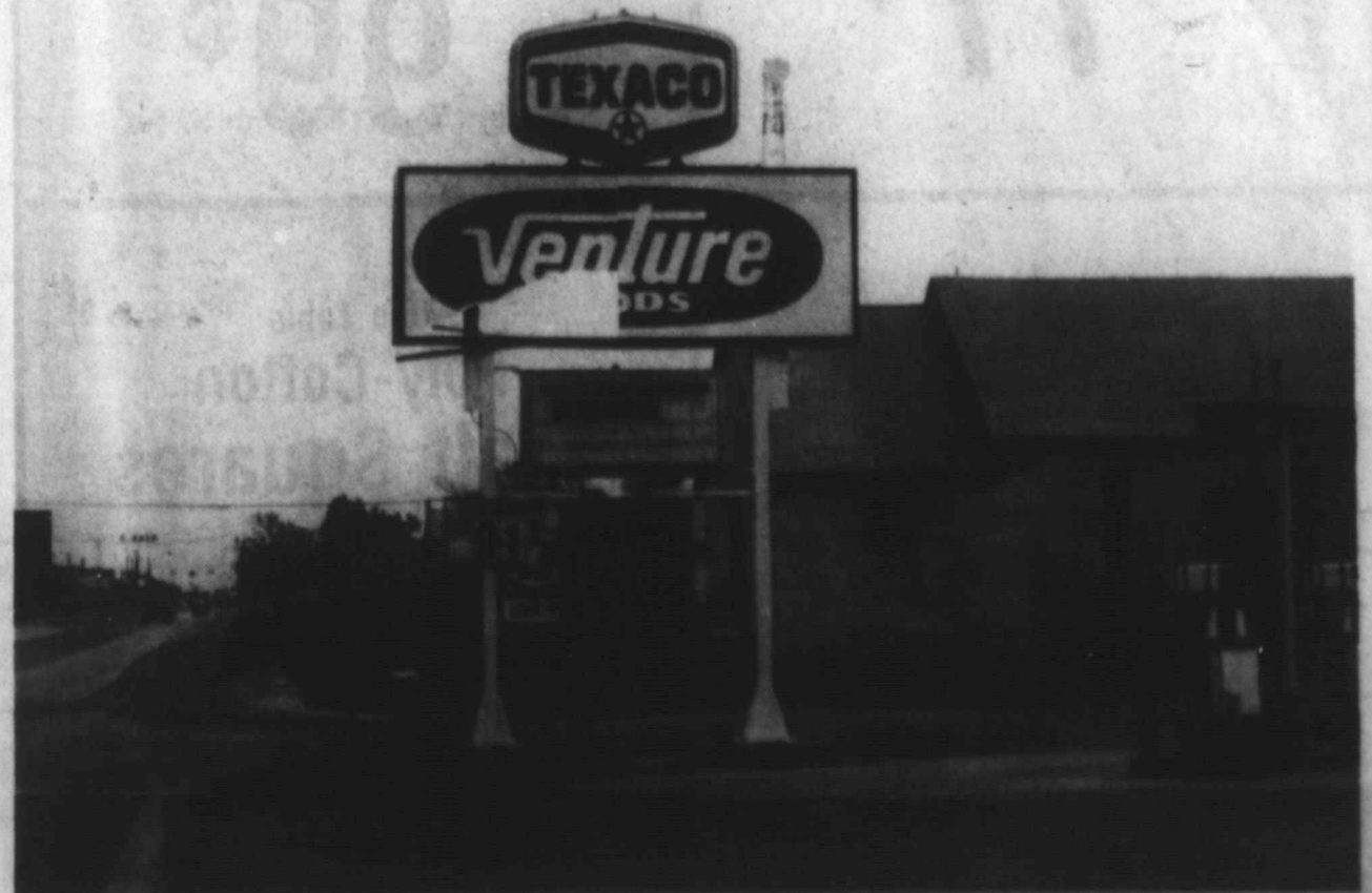
WIND DAMAGE --Summitt Venture Foods sign was partially blown away by the high winds in the area Monday, when gusts reached about 60 mph. Some fences were damaged also in Tahoka and elsewhere in the county. (LYNN COUNTY NEWS PHOTO)
