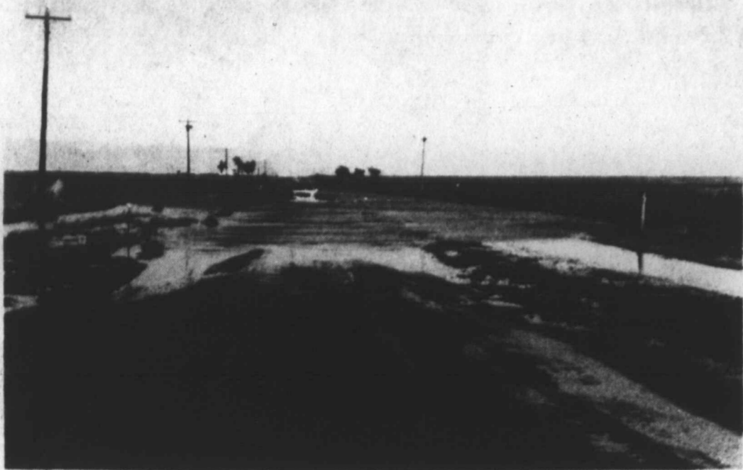
ROAD FLOODED --Recent rains inundated several roads in the county. This photo shows a road two miles west of New Home that was impassable for three days. (Photo courtesy of Joe D. Unfred)
