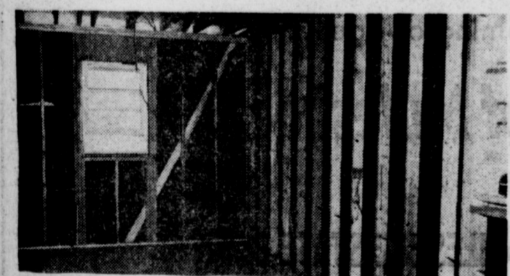
MORE secrets of Avinger superiority . . . 2 x 4-inch uprights and 2 x 6-inch ceiling joists on 16-inch centers. And it's ready for beautiful hardwood flooring.
