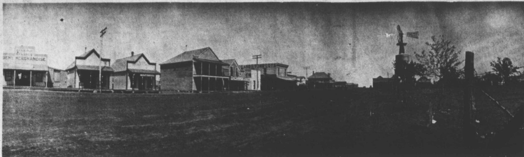
WEST SIDE OF SQUARE in Tahoka as it appeared in 1910. Some of the buildings identified above are Wells and Welcher General Merchandise on the extreme left and Charley Brown Real Estate. In center of picture is the W.C. Cowan Bldg., Howell and McGill Drug Store and
