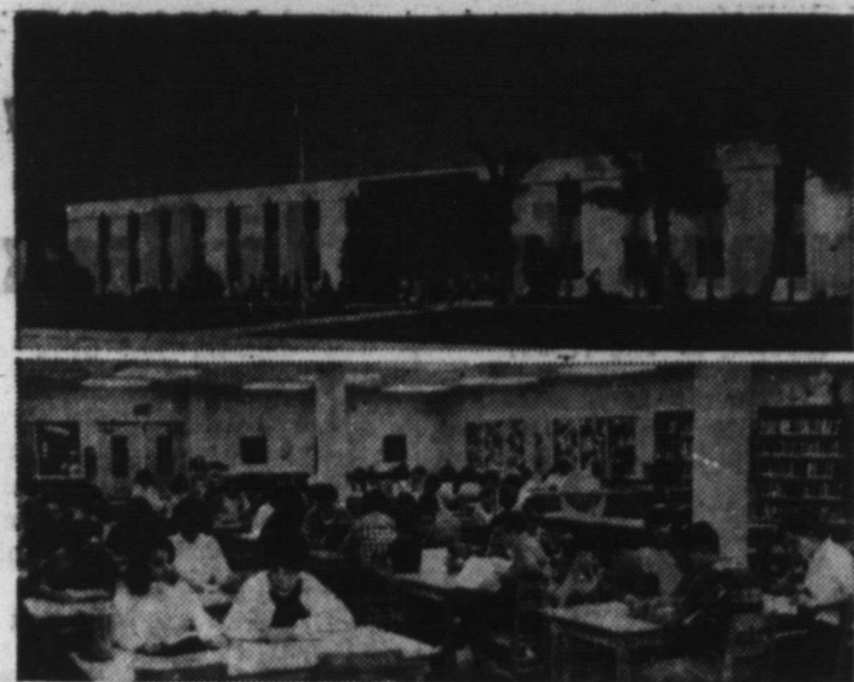
MIAMI CORAL PARK Senior High School in Florida is one of five school buildings in the Miami area for which fallout shelter was especially designed. The library (lower photo) is part of a central core of rooms protected from radiation on all sides and above by corridors or classrooms and providing shelter space for 1,850. Small windows and an attractive exterior baffle wall (top photo, at center) shielding the main entrance corridor from radiation are added fallout-protective features. The technique of providing a radiation-shielded central core area containing the school's service facilities has been praised by school officials. Miami Coral Park is one of 34 structures cited in "New Buildings With Fallout Protection" (TR-27), a newly issued publication of the Defense Department's Office of Civil Defense.
