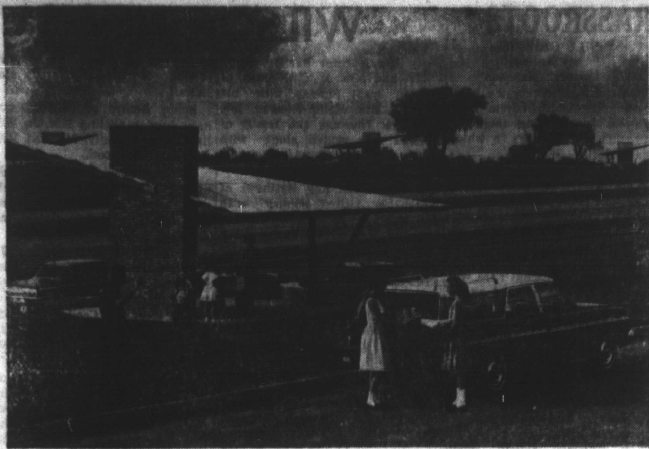
The Interstate Highway System in Texas is being blessed with large, elaborate Safety Rest Areas for the safety and convenience of Texas travelers. Motorists can now relax and refresh themselves in the first of these rest areas (roadside parks) designed and built on the Interstate Highway System in Texas. This new rest area contains eight arbors equipped with five places for family cooking, incinerators, fire wood, and big spacious tables and benches for picnicking. The "park" lies on a small knoll ten miles east of San Antonio on Interstate Highway 10 and was formally dedicated May 29.
