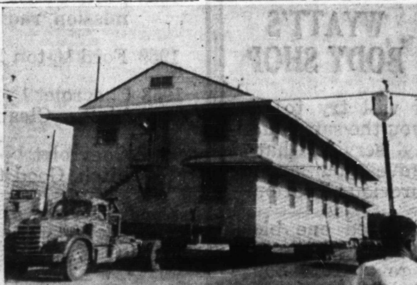
BOYS RANCH BUILDING is pictured above as it came down main street recently headed for the ranch site on the old C. W. Slover farm, now owned by Jack Miller, executive director, who has leased 50 acres to South Plains Boys Ranch and option to buy. The building is a former Lubbock church education building which will be remodeled as a dormitory for the boys.
