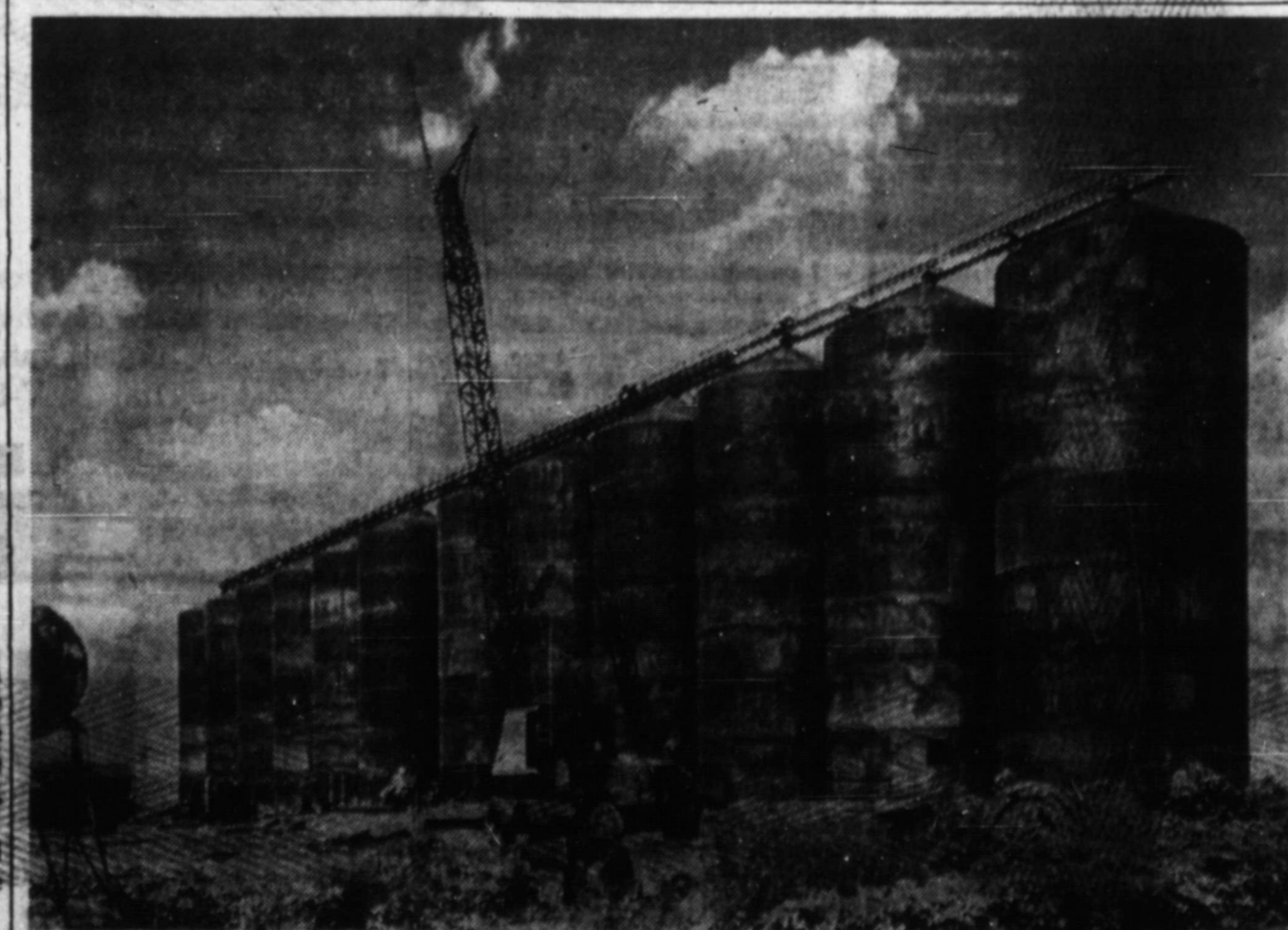
NEW GRAIN STORAGE tanks, shown above, being installed on Santa Fe trucks by Goodpasture Grain & Milling Co., will be completed in time for the maize harvest. The 12 tanks replace the old burned elevator and will furnish storage for about seven million pounds of grain. Completion of this project is expected by August 15. (Photo by Finney)
