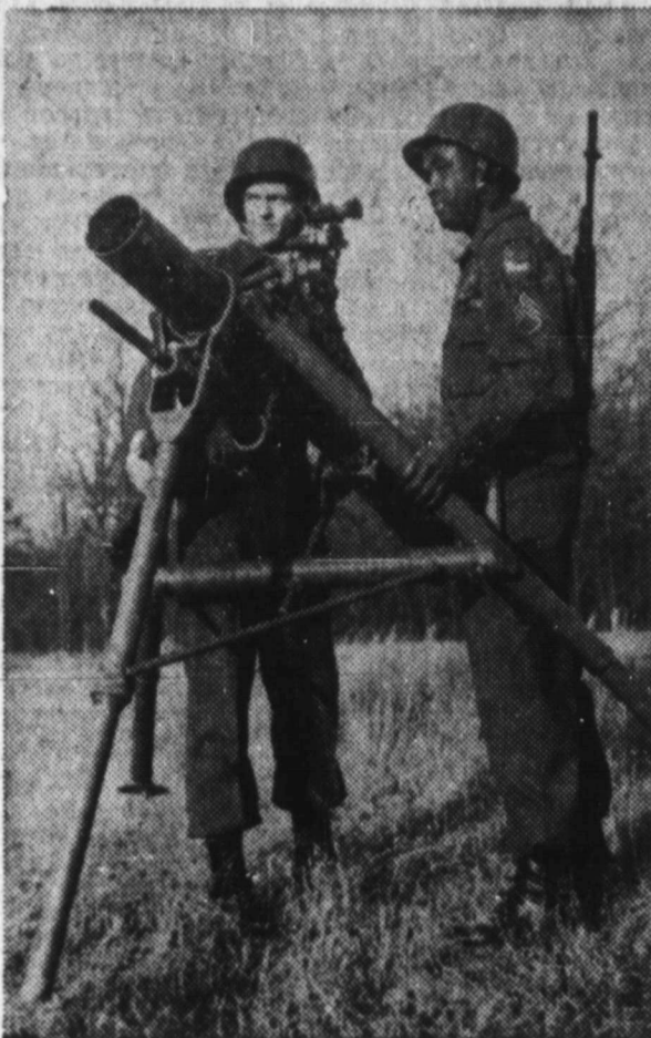
ARMY'S LATEST—mobile weapons system, the DAVY CROCKETT, displayed at Fort Benning, Georgia, during PROJECT MAN, a demonstration recently held to focus public attention on Modern Army Needs. A hand or portable weapons system, DAVY CROCKETT is capable of firing atomic or conventional warheads in support of Army's front line pentomic battle groups. The weapon is scheduled for production in Fiscal Year 1961.
