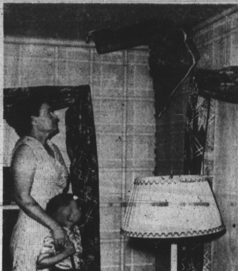
TIMBER THROUGH WALL—Mrs. C. M. Meador, whose husband works for Gilmore & Jaquess, and son, Eddie, 5, survey damage done to home near old light plant when a two-by-four board was driven through the corner of a room by the tornado of May 24. Mrs. Meador and son were in a storm cellar when the tornado struck. (Avalanche Photo).
