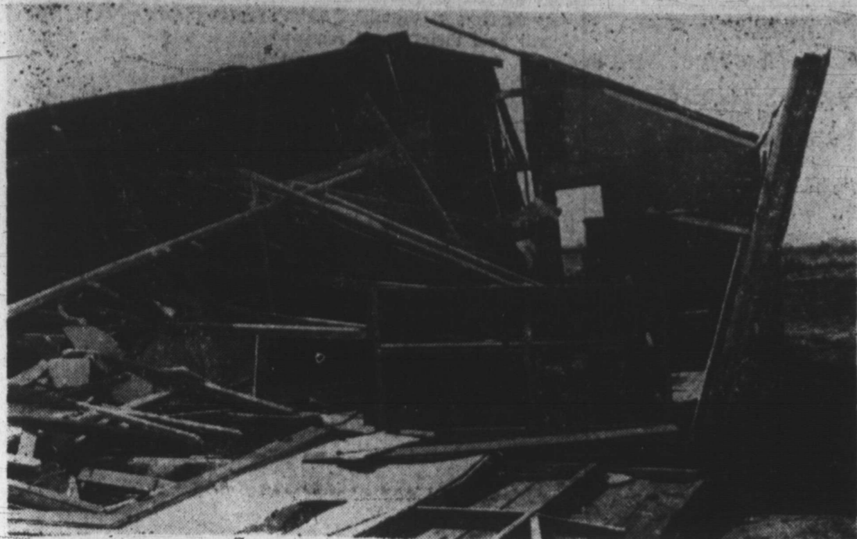
CHURCH WRECKAGE—Shown above is the Antioch Baptist Church following the Tahoka tornado, with part of the pews and the piano, the only part of the building and furnishings not destroyed.
