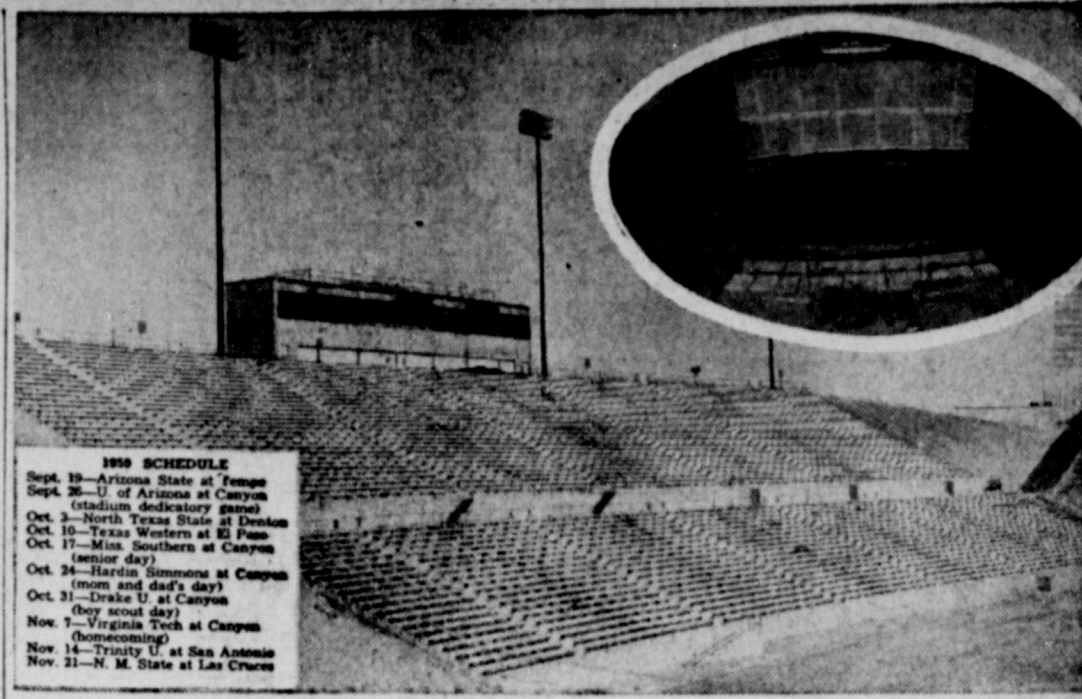
WEST TEXAS STATE'S BUFFALOES will christen a modern 20,000 seat football stadium this fall with area's first "major" schedule. The Buffs will meet Arizona, Mississippi Southern, Hardin-Simmons, Drake and Virginia Tech in that order in the new plant, which is located two miles north of Canyon and 13 miles south of Amarillo on the E-way. Above is a close-up of the west stands and the inset shows an aerial view looking from the East. An open house at the stadium is scheduled from 4 to 6 p. m., Sunday, Sept. 13.
