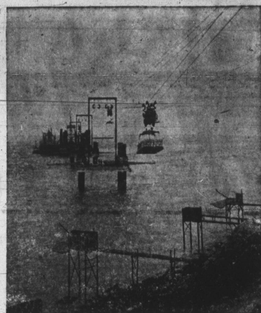
HIGH-FLYING CARGO—A skycar transports 20 tons of Army supplies at a 35-mile-an-hour clip over an aerial skyway to a safe discharge atop a rocky cliff face in France. Cargo ships are independent of port facilities when they tie up to a movable DeLong pier. Retractable piles allow submerging for concealment.
