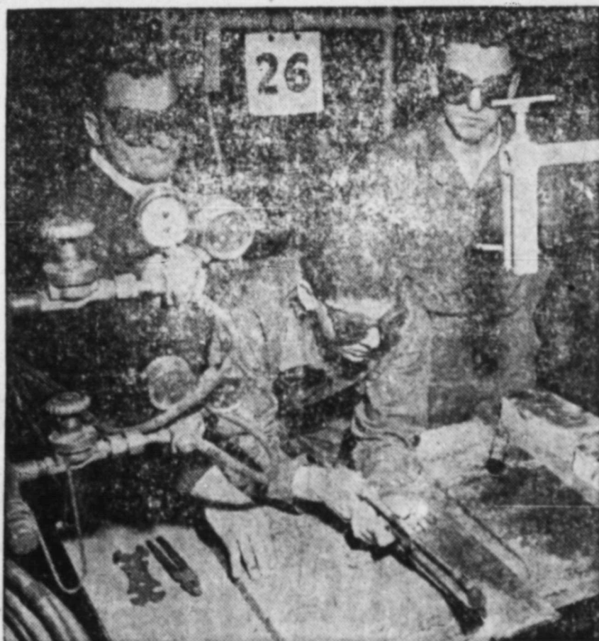
FLAME-CUTTER—Private William A. Wilson of Syracuse, N.Y., a Reserve Forces Act enlistee, is learning to use an oxygen-acetylene torch during the last phase of his six months' active duty at the Army Quartermaster Center, Fort Lee, Va. Mr. Joe P. Richman, the instructor, is at left, and Private Landon G. Edwards, also from Syracuse, is at right. Both will find this skill useful on job-hunts.
