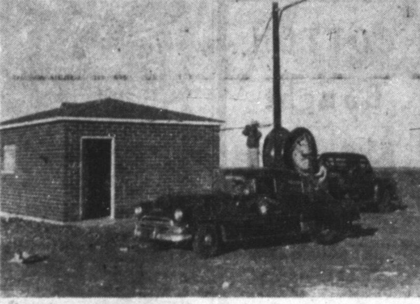
TELEPHONE EXCHANGE—Pictured above is one of the buildings which will house six automatic unattended central exchanges of the Peka-Lambro Rural Telephone Cooperative in Lynn county, in which equipment is now being installed.
