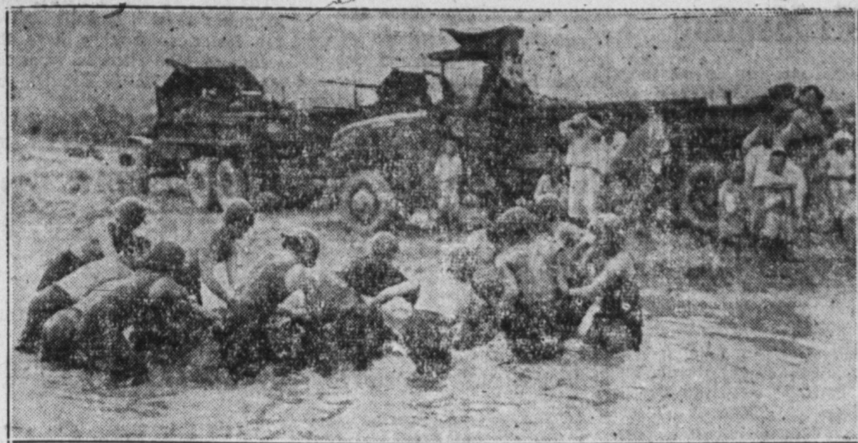
BATTLELINE STRUGGLE IS NOT ALL SHOOTING—U. S. Army Engineers use two-wheeled native cart to remove boulders from Korean river bed to open a ford for the advance of American motor vehicles.
