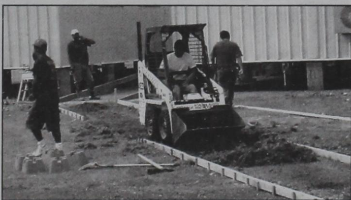
Workers at DeShazo Elementary prepare new walkways to the temporary classrooms.
