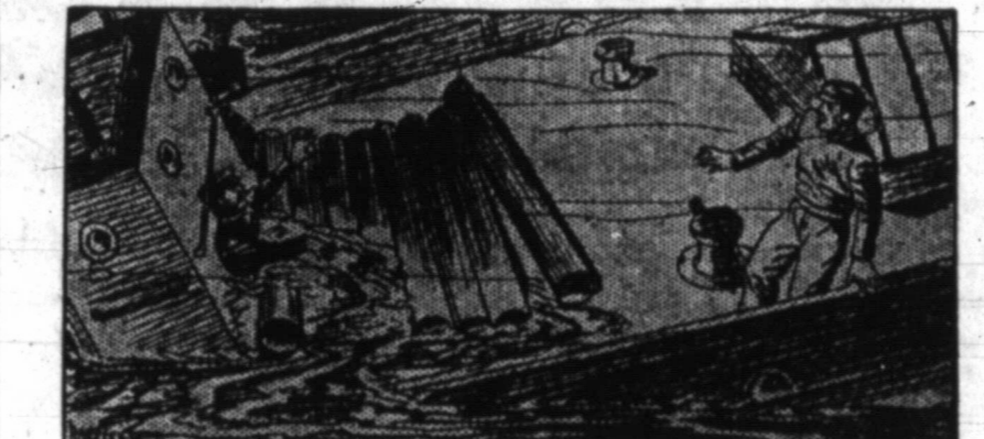
Williams Was Pinned to the Deck House.
