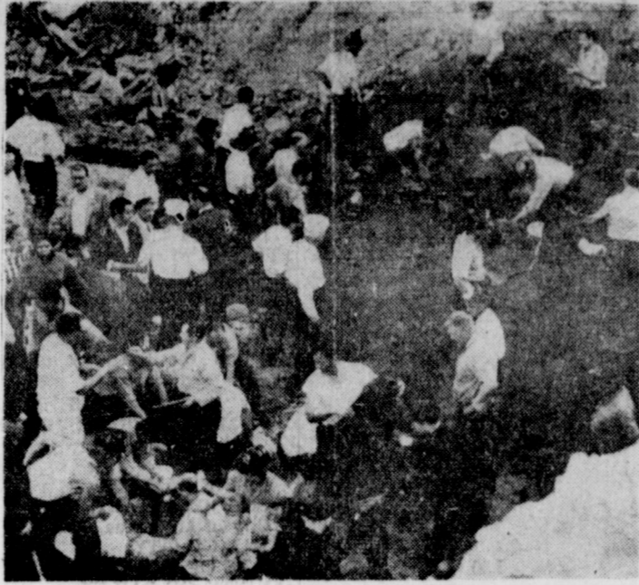
CAVE-IN TRAGEDY — 6 CHILDREN DEAD — This is a general view of the excavation site in New York where six children were killed when they were buried under tons of earth while playing in 25-foot deep pit. Rescue workers can be seen working with pulmotors over one of the victims, a little girl. An investigation is now under way to determine responsibility for the apparently unguarded project.
