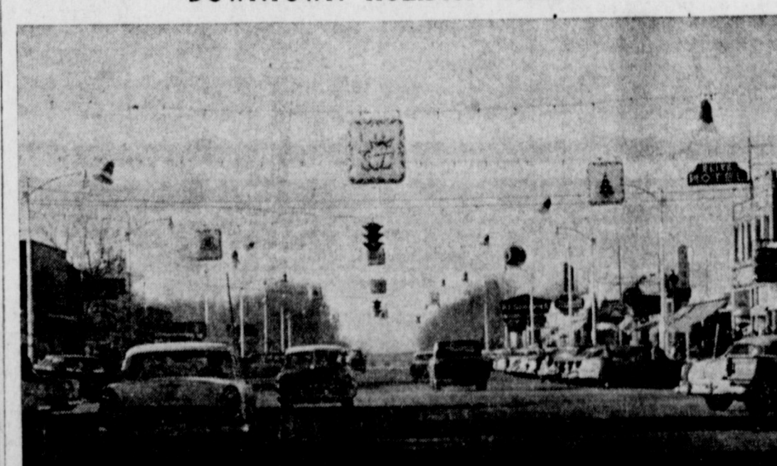
BEFORE THE WINDS CAME, Main street was decked out in new holiday decorations. After the high winds Saturday and Tuesday, several of the decorations like the one in the center shown, here, blew away and have not been recovered.
