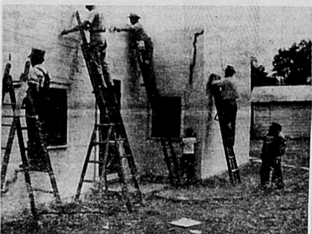
HARD AT WORK — Owen Thompson, Charles Reeves, Fred Hart, Jay Reeves and Lonnie Ray join hands in scraping old paint off walls of Chamber of Commerce doctors clinic. The group of volunteers are working to get the building in top condition for the doctor the Chamber of Commerce is seeking for Baird. Inspecting the work is Raymond Young, president of the Baird Chamber of Commerce.
