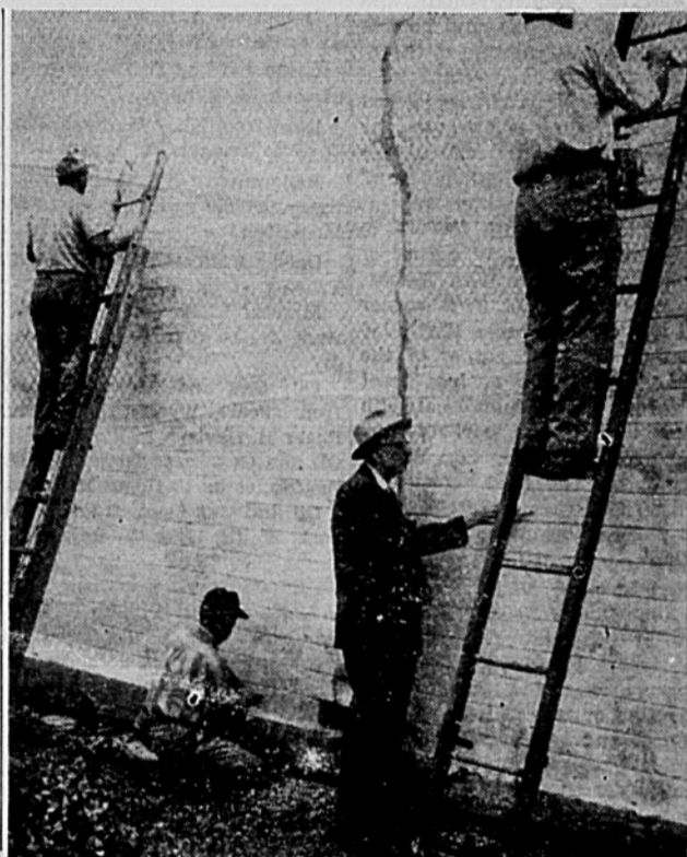
BANK PRESIDENT JOINS IN WORK — Bob Norrell, president of the Baird First National Bank, joined volunteer workers Saturday in working on doctors clinic purchased recently by the Chamber of Commerce. Working along side Mr. Norrell are Fred Hart, Rancher and oil man; Charles Reeves, Lumberman and Lonnie Ray, retired auto dealer.
