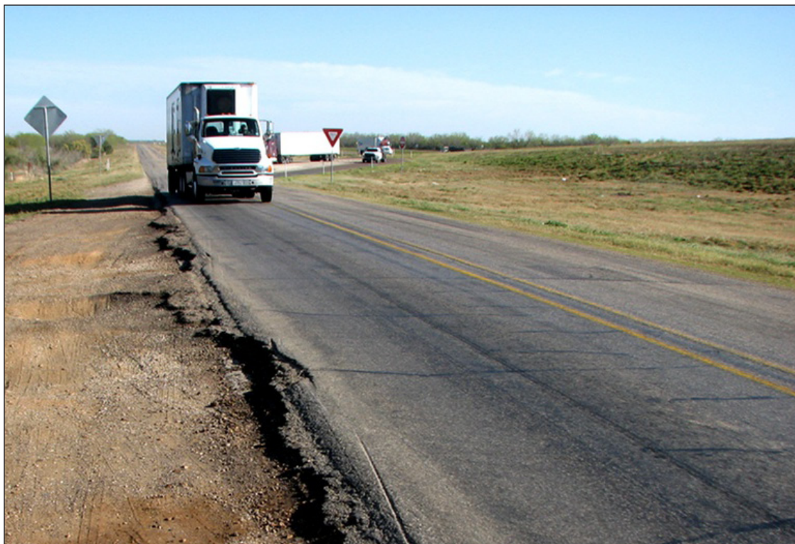
TEXAS DEPARTMENT OF TRANSPORTATION | SUBMITTED PHOTO A NATURAL GAS DRILLING BOOM in the South and West Texas areas are straining the area's rural roads as more than 1,000 loaded trucks are needed to bring a single well into production.
