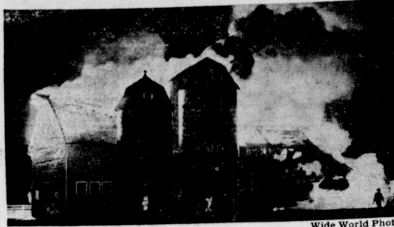
The labor and production of many months went up in flame as fire destroyed this Indiana barn and its contents, including 700 bushels of corn and 100 tons of newly harvested hay. If the moisture content of hay is too high when it is stored, fire by spontaneous ignition often results.
