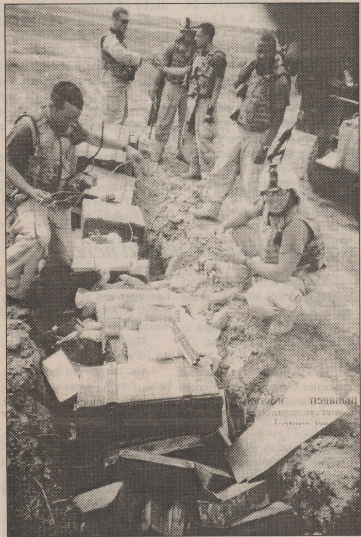
JOSH ARAUJO'S 8-MAN TEAM sets up demolition of weapons caches outside the town of Afak, Iraq. Submitted Photo
