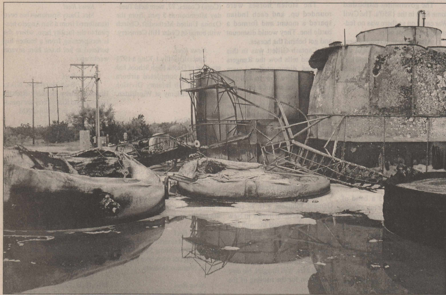
THREE MELTED Fiberglass tanks appear to float on a sea of water and foam at the Wilson Disposal Unit on Pandale Road. Lightning struck two tanks at once, causing the early morning fire June 15.
