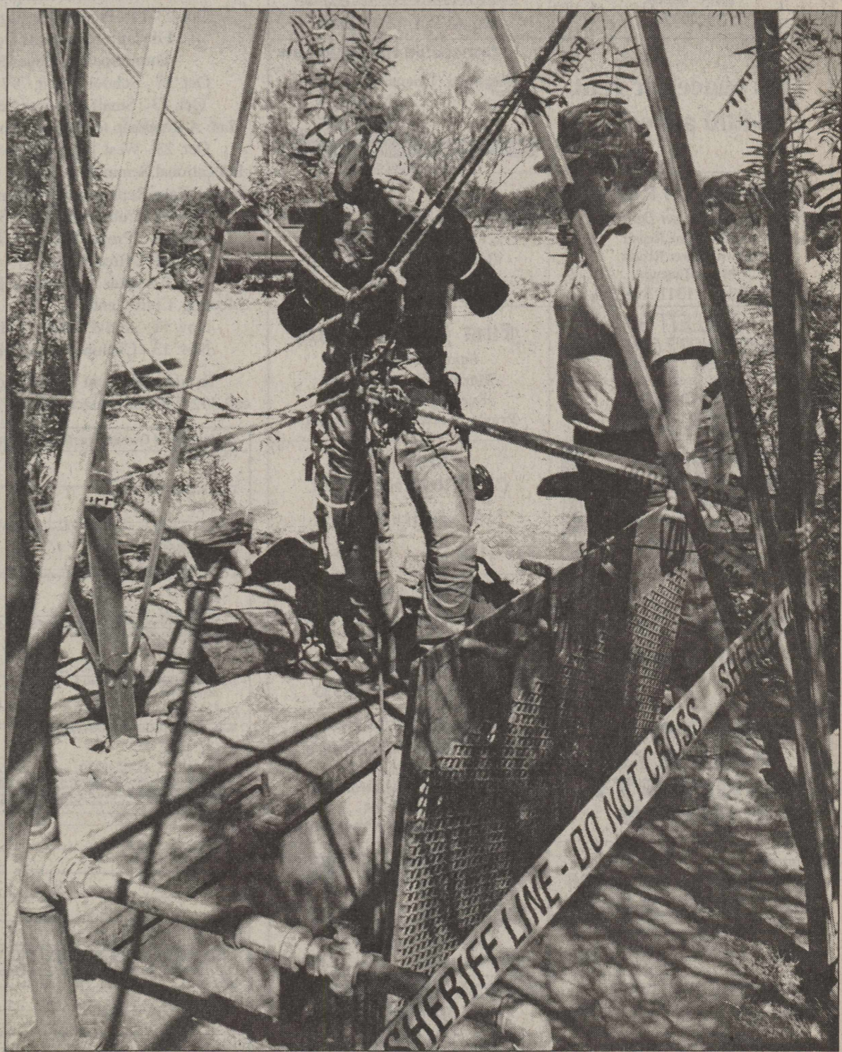
MEMBER OF THE AUSTIN CAVE RESCUE TEAM prepares his rigging before he begins his trip down the narrow drop of 125 feet into 0-9 Well Cave. The rescuers had to coordinate signals between the surface group and the underground group before the body was hoisted to the surface. photo by Scotty Moore
