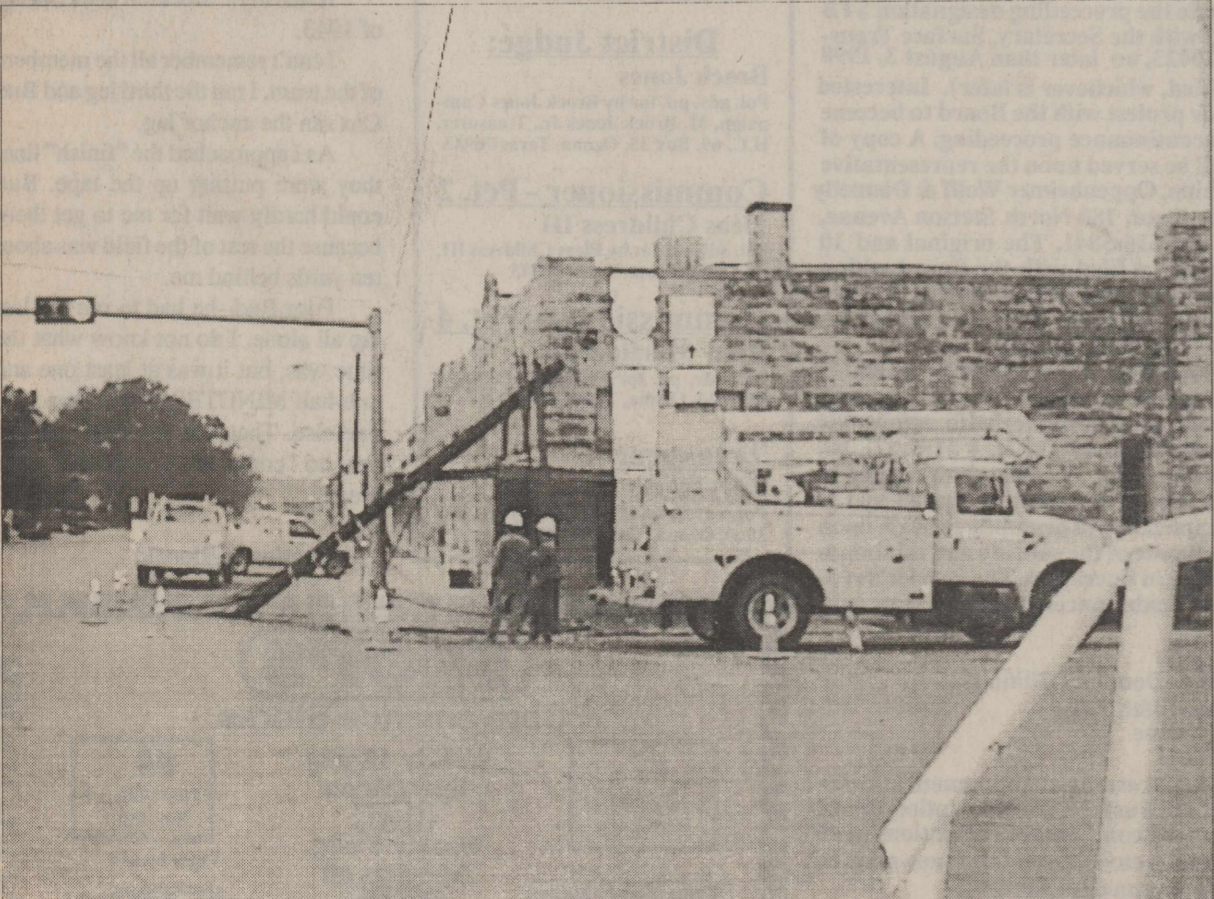
A WIPED OUT UTILITY POLE at the intersection of Highway 163 and 290 brought everyone out nice and early on Thursday, June 5. At presstime the only clue of 5:47 a.m. hit and run accident was green paint left on the pole.
