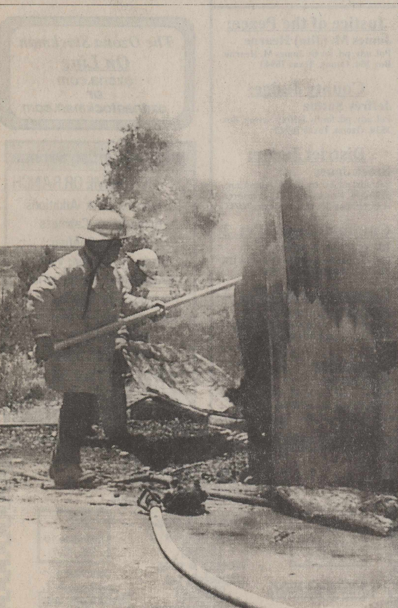
OZONA VOLUNTEER FIREMEN battled a blaze on Monday in a storage building belonging to Deene Holden at the Hillside Estates just north of town. DigiCam Photo by Susan Calloway
