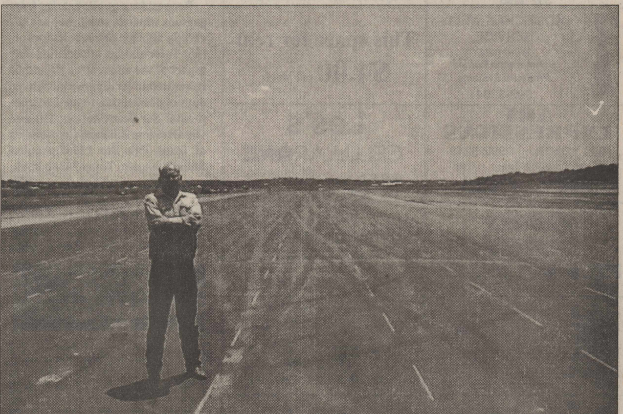
JIM HEARNE stands in the middle of the new runway at Ozona Municipal airport. The construction, which began in October of 1997, is nearing completion. DigiCam Photo by Scotty Moore
