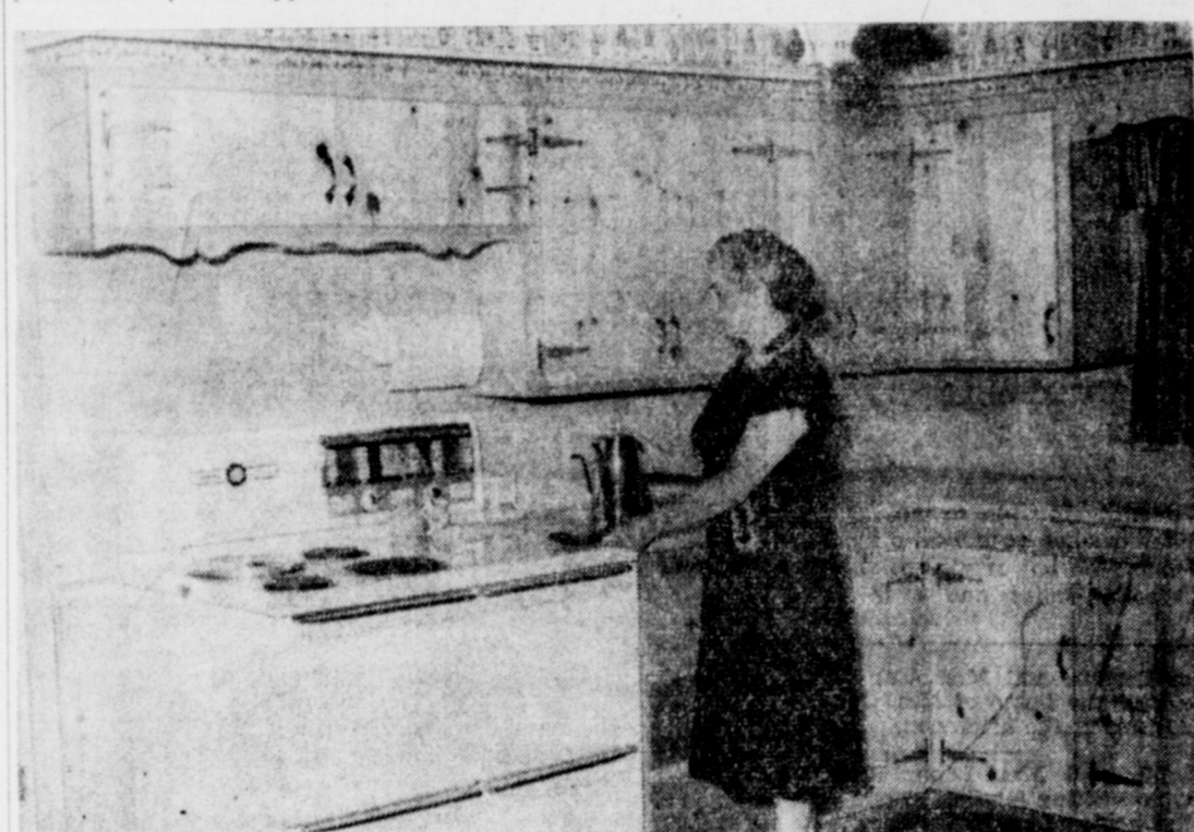
MRS. W. T. ANDREWS is shown here in the new kitchen of her home. The kitchen and dining room were added on to the house after the Andrews bought it. (Staff Photo)
