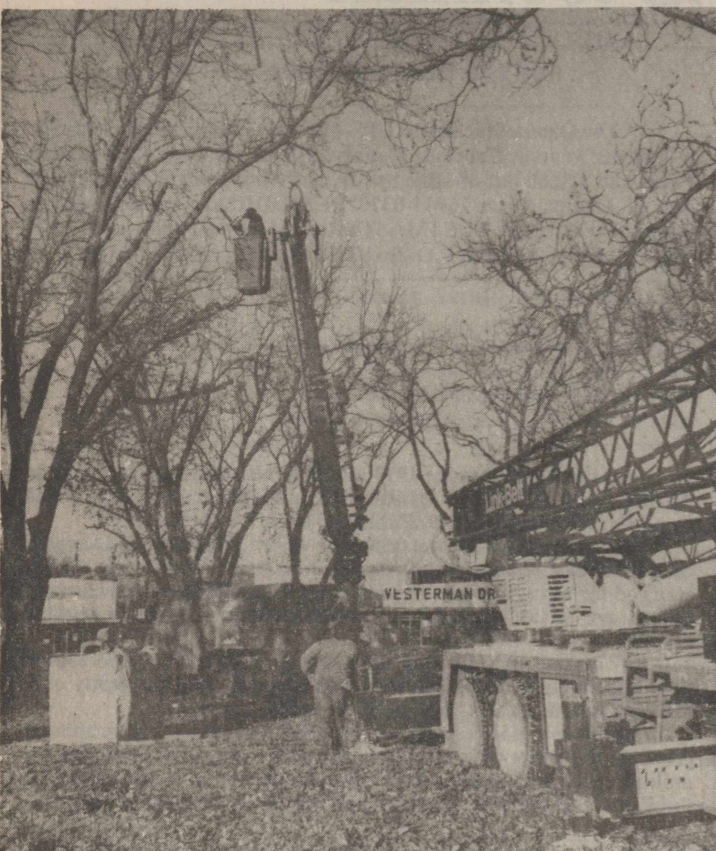
BRANCHES ARE BEING TRIMMED before placing the granite base to the Heritage statue (left foreground) in the center of the square. The completed statue will be brought to Ozona by mid-January. The inscription on the base reads: "The Tie That Binds by Judy Black December 1996 A Heritage Appreciation Sculpture Dedicated to the Pioneers of Crockett County". photo by Scotty Moore
