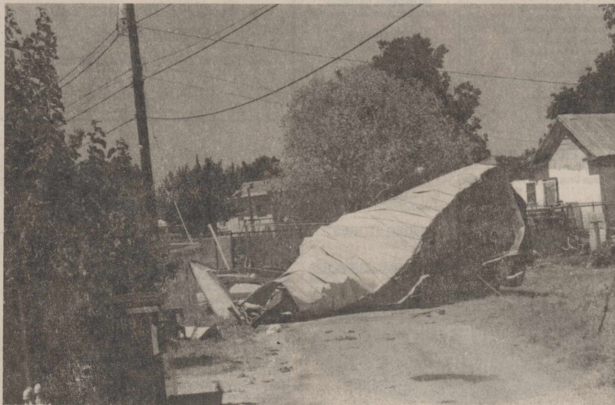
THE DIAZ HOME in the 1800 block of Walnut Street had this storage building lifted over the fence and hurled into an alley during a severe windstorm Saturday night.
